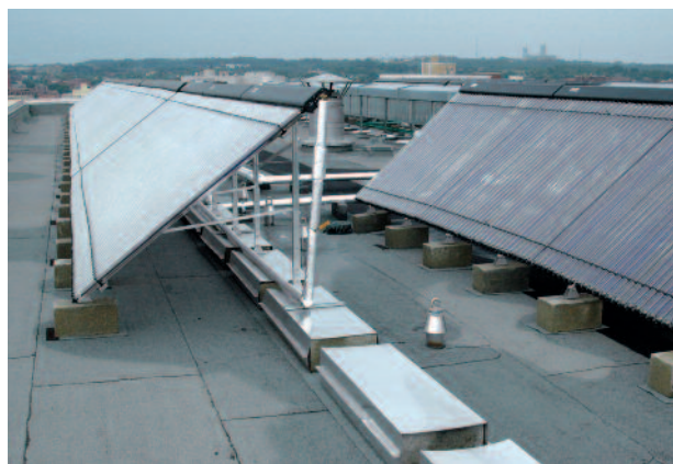
Figure 29: Collector system ballasted with concrete blocks
