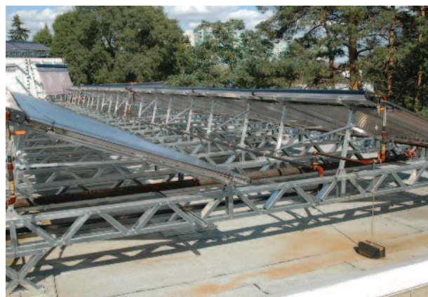
Figure 32: System utilizing a grille with minimal roof penetrations to attach to the grille of the building – the weight of the system reduces the number of penetrations required
