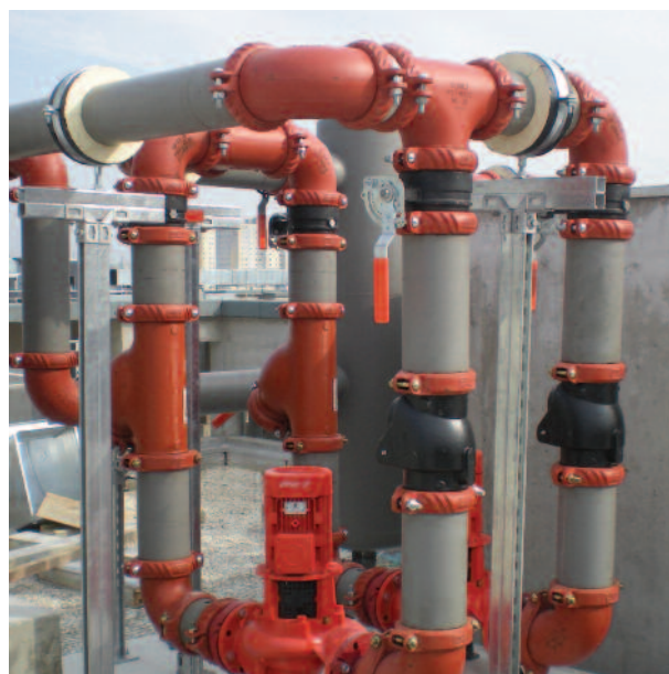
Figure 27: Pump system with Victaulic fittings
