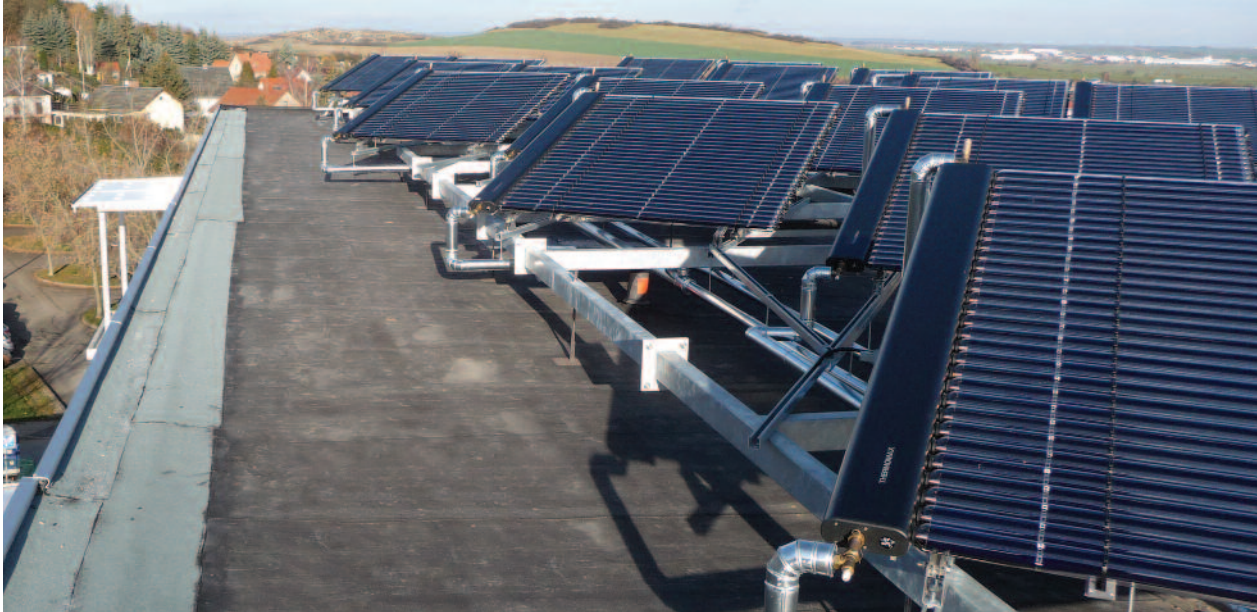
Direct Flow System, Apartment Building, ARNSTADT, GERMANY
