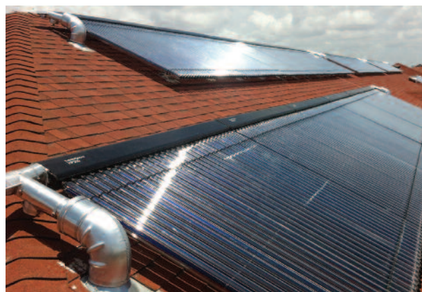
Figure 30: Here the collectors have been attached to the roof with standoffs that are individually sealed. Each collector has four attachment points
